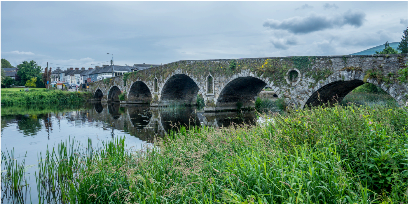
Above: Goresbridge town in the background and Gore's Bridge, centre, crossing the Barrow River. Our Ryan ancestors would have crossed this many times. Goresbridge is a village only a few kilometers from Borris village. This bridge, the "new" one, dates to 1756. The bridge was the site of the Battle of Goresbridge during the Irish Rebellion on June 23, 1798.
